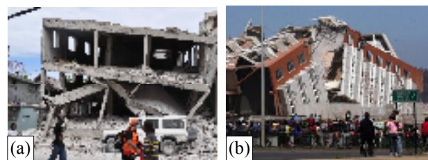
Figure 2: Buildings Damaged by the 2010 (a) Haiti and (b) Chile Earthquakes
