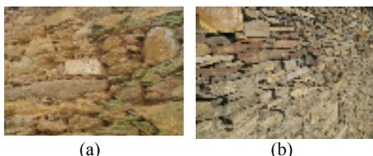
Figure 3 – Joint in schist masonry: (a) With earth mortar; (b) Without mortar.
