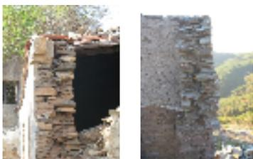
Figure 2 – Two leaves walls without connection.
