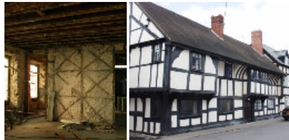
Figure 1: Typical half-timbered structures: a Pombalino wall in Lisbon (left) and a half-timbered building in Herefordshire, England (right)
