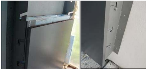
Figure 2: Retrofit module installation on the support structure
