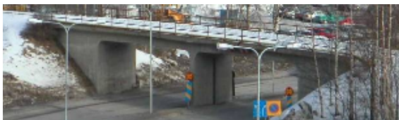
Figure 5: Örnsköldsvik Bridge (Sweden)
