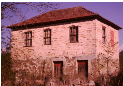
Figure 1: Masonry building in Monção, Portugal
