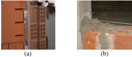
Figure 2: Infill solutions: (a) model one with a double leaf unreinforced infill; (b) model two with a single leaf reinforced infill
